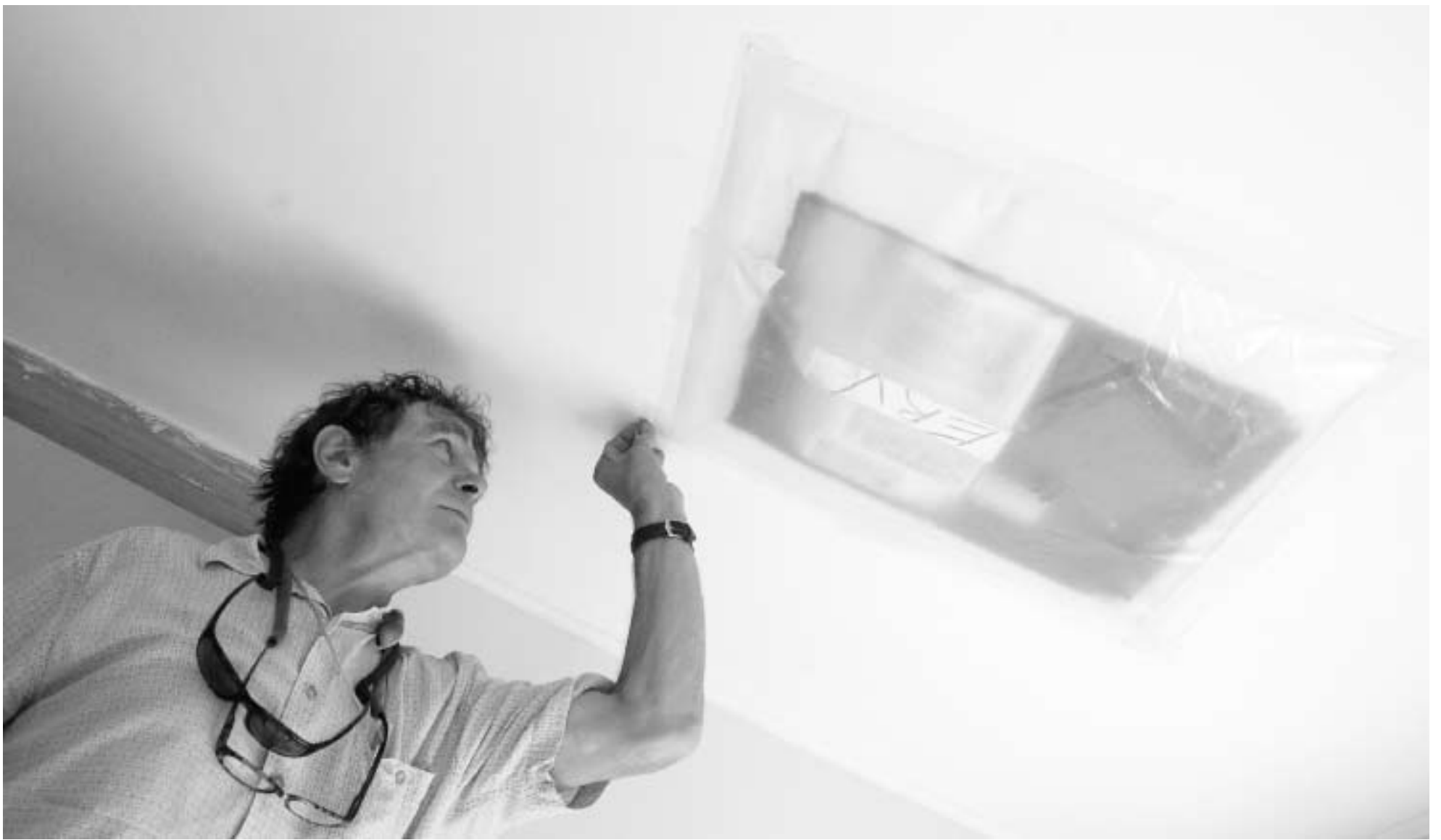
Contractor Terry Nordbye inspects the ventilator, which circulates air throughout the sealed Passive House, remodeled by CLAM. Photo by Sasha Portis.
